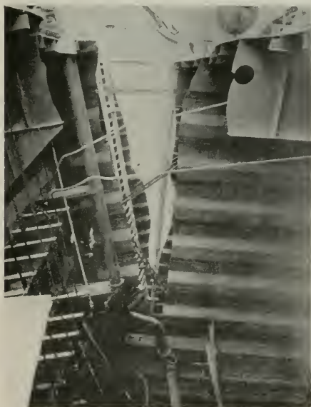
Inboard view of fracture of Schenectady showing clean break of all structural members.
